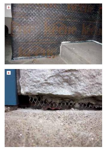
to drain to the outside from behind the brick. To create a drainable system, I always use a rainscreen material, such as Keene Driwall (keenebuilding.com), which is shown in the photos for this job. Recently I have been using MTI Cavity Gravity (mtidry.com), which was developed for brick walls but also works with EIFS and ACMV. It stays rigid, which makes applying the lath easier and helps to maintain an even thickness for the scratch coat.
